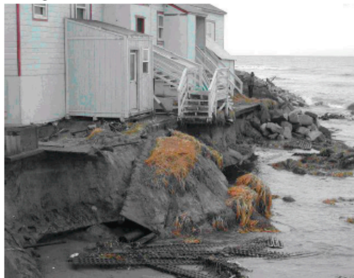
Coastal Storm Activity Undermines Foundations in Western Alaska (USACE,
