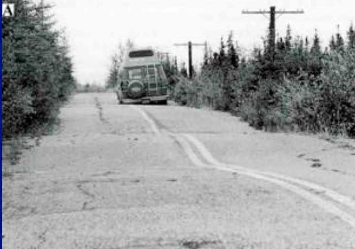
Alaska Road Heaves
