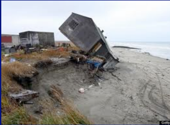
Coastal Erosion, Alaska
