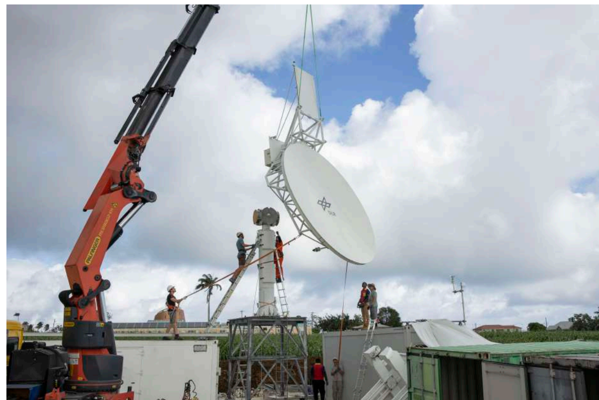
Installing the Poldirad C-band radar on Barbados
